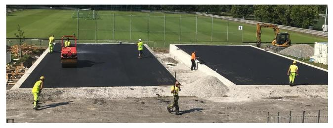
Drainpipes from "the concrete box" outside that leads the rain water out smoothly. Asphalt 1-2 layers before installation of the sports grass. Asphalt helps to speed up the drying process after the rain.
