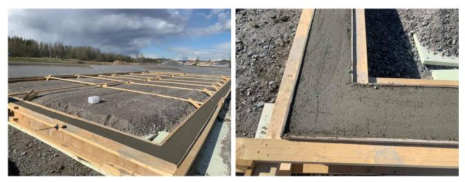
Concrete foundation 30-40cm wide based on the outdoor measures of the Padel court. Court size inside of the structure is is 20000mm x 10000mm and space needed for the installation of Premium Panoramic Court is minimum 20500mm x 10500mm. Inside measures of the concrete structure are 20000mm x 10000mm.
